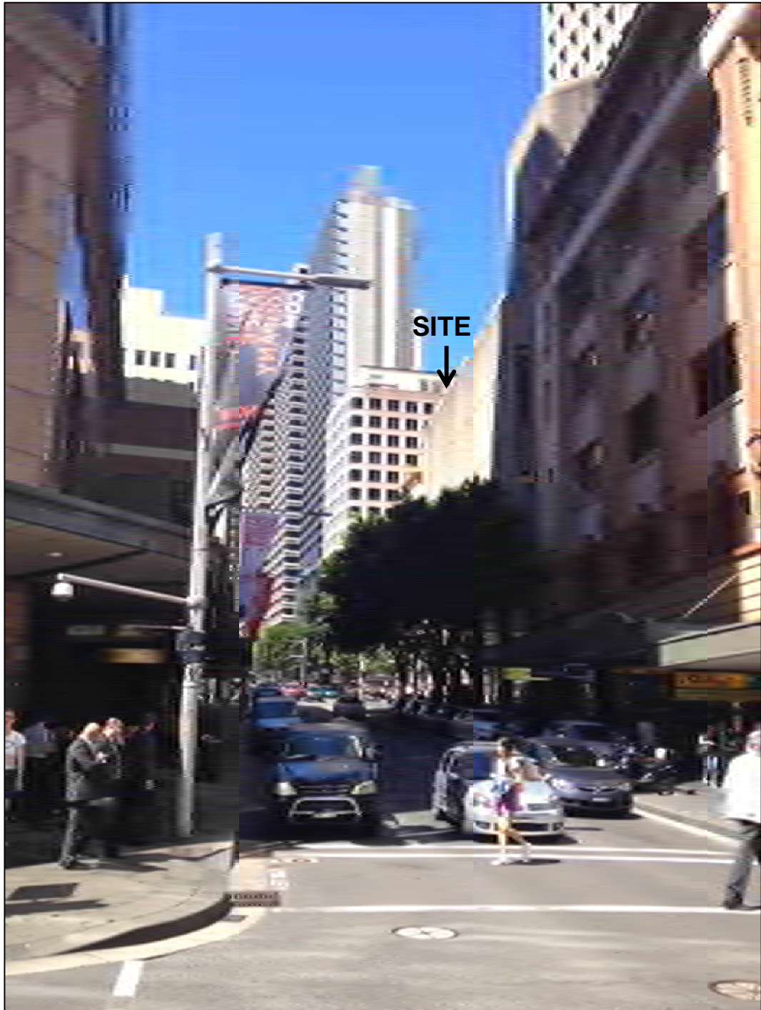
Figure 5: View looking eastwards along Liverpool Street towards the site
