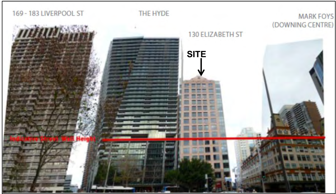
Figure 26: Lack of established podium on adjacent buildings on Liverpool Street, and location of podium interpretation zone to reflect height of the adjacent State heritage listed Mark Foy Emporium building
